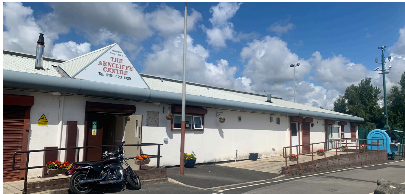
Figure 7 shows a photograph of the current Arncliffe Centre
